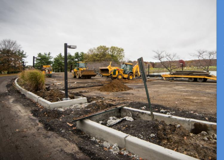
As of November, Somerset is putting the finishing touches on the Grand Entry Piazza – the building's front entryway for guests and visiting prospective tenants. The company is fixing the lot's decades-old base, installing new curbs, removing old storm grates, and repaving the lot. The new entryway holds space for over 100 cars.
